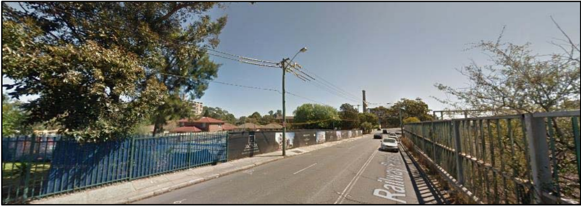
Figure 12. Northern frontage of the site to Railway Parade looking north-west (Source: google.maps.com.au)
